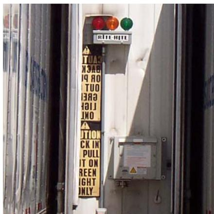
**Figure 3-3: Installed trailer connection with new lighting fixture**
