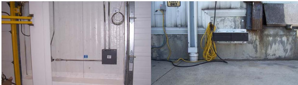
**Figure 3-4: Electrical wiring for eTRU connection**      **Figure 3-5: Protective bumper for eTRU connection**
