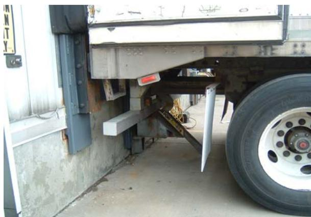
**Figure 1-4: Trailer secured to warehouse dock with dock safety system**
